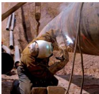
Welder working on the Chad-Cameroon pipeline.
