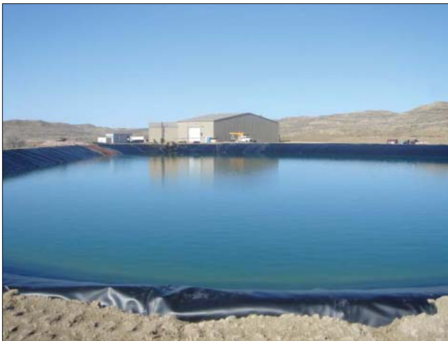
The CBM water-treatment plant currently has a 30,000-b/d capacity. In the foreground is the inlet pond (Fig. 1).
